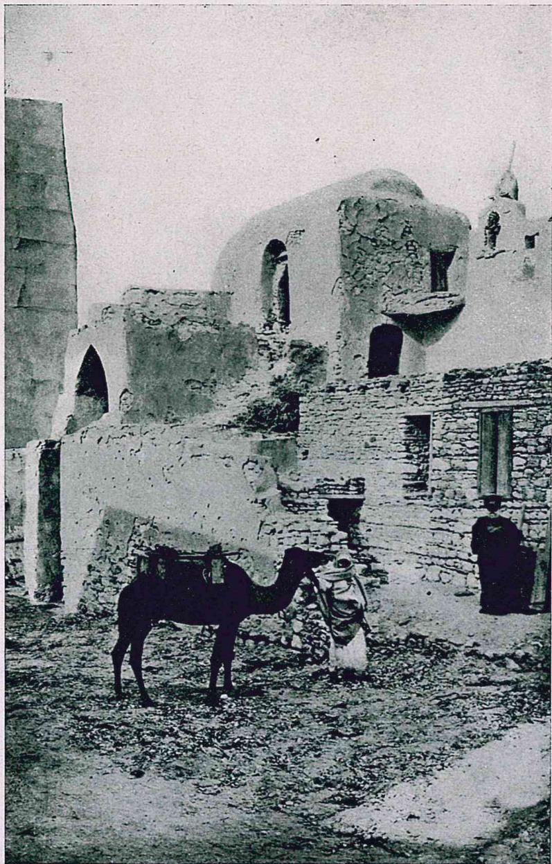
Gatehouse of Dair al-Baramûs
